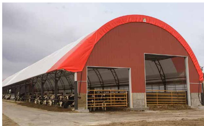
A 40-foot-wide hoop building is used for feeding cattle.
